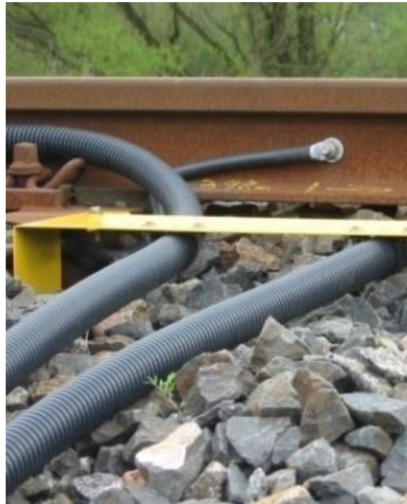
Rail foot cable branch with divisible corrugated tube
